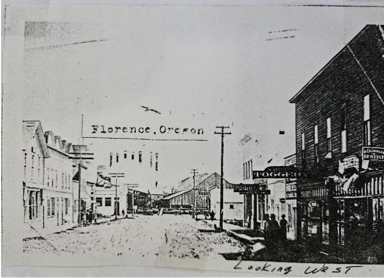
Main street (now Bay Street) Florence in the late 1800s.
